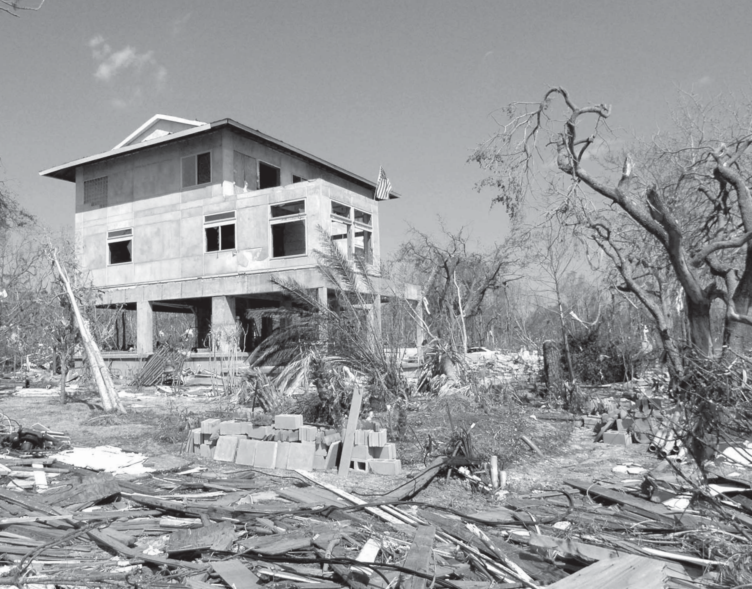
THE OWNER OF THIS HOME IN PASS CHRISTIAN, MISSISSIPPI, WAS IN THE PROCESS OF BUILDING A STEEL-REINFORCED CONCRETE HOUSE USING MANY FEMA BUILDING STANDARDS. THE HOUSE WAS THE ONLY ONE LEFT STANDING AFTER HURRICANE KATRINA PASSED THROUGH THE AREA.
